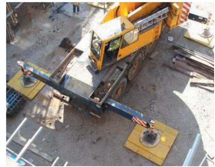
The Contractor must provide a hardstanding of adequate bearing capacity to withstand the anticipated worst case outrigger loadings, as will be notified by the Company Representative (the visiting supervisor of the precast company). All those involved in the accommodation, planning and implementation of lifting operations must understand the issue of outrigger loadings and the careful consideration required to ensure the precast concrete components can be lifted into position in a safe manner.
